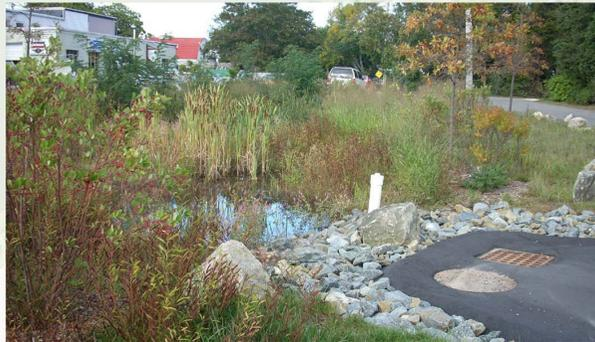
Constructed wetlands offer a more naturalistic approach for stormwater remediation, as constructed in Orleans, MA.
