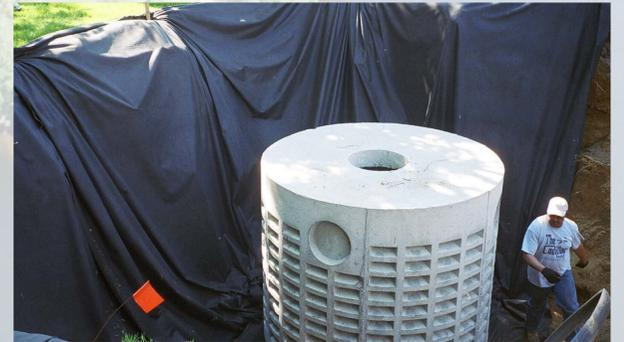
Where field conditions allow, traditional sub-surface leaching is a proven approach for stormwater treatment.
