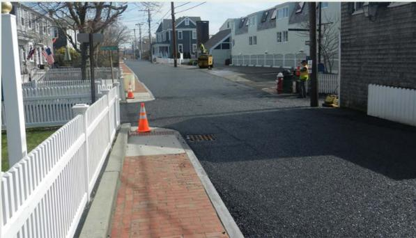
Porous asphalt installed in Provincetown, MA has virtually eliminated beach closures due to stormwater runoff.
