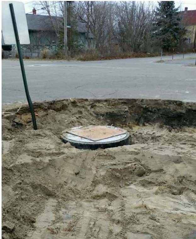
Figure 3. Existing drainage structure prior to being adjusted to meet new grades.
