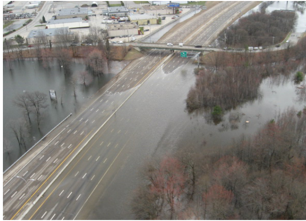
The Pawtuxet River flooded Interstate 95 on March 31. Photo: R.I. Dept. of Environmental Management.
