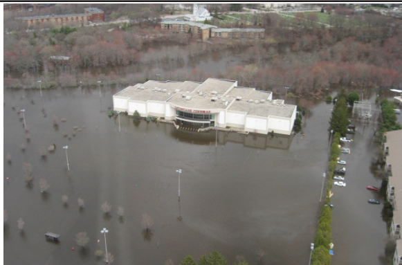
Showcase Cinemas in Warwick, R.I., was built on a floodplain which was flooded in March. Photo: R.I. Dept. of Environmental Management.
