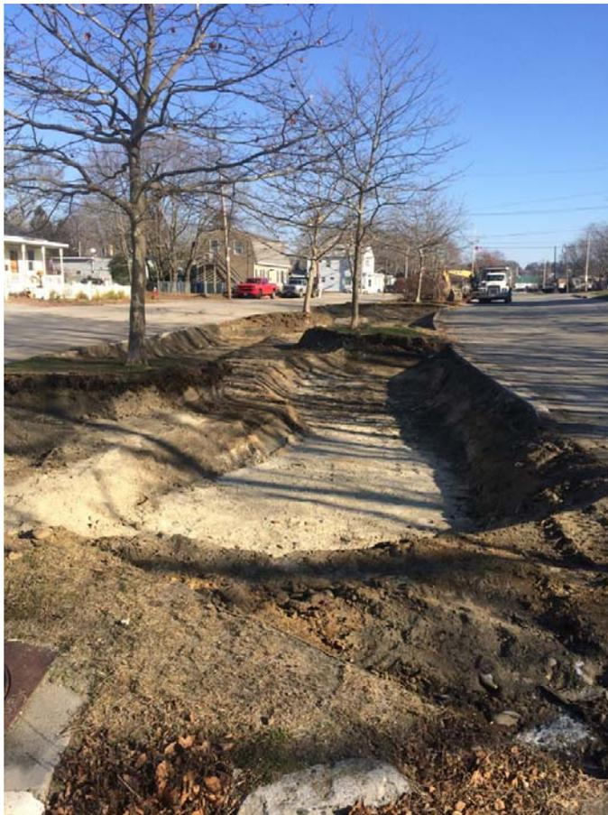
Figure 1. This photo shows one of the bioretention locations with top soil removed and rough grading to sub grade material.
