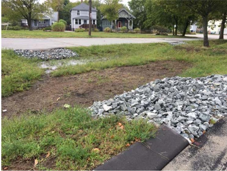
Figure 2. Bio-Retention basin with bio-retention media and stone erosion controls.
