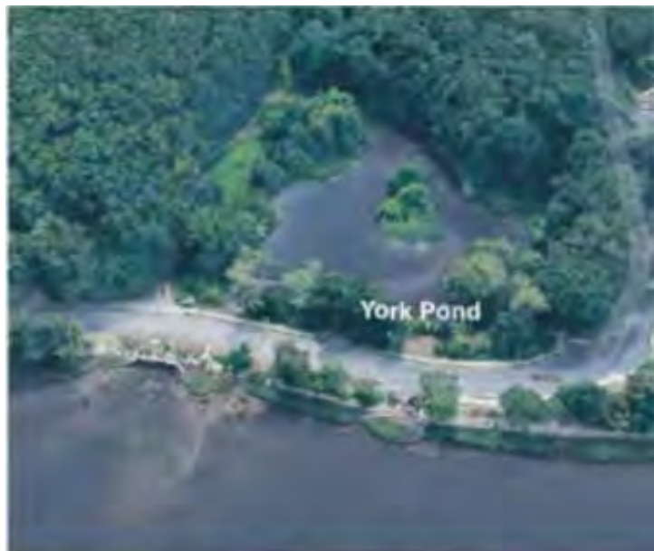
York Pond discharging to the Seekonk River. Photo Credit: Groundwork RI.
