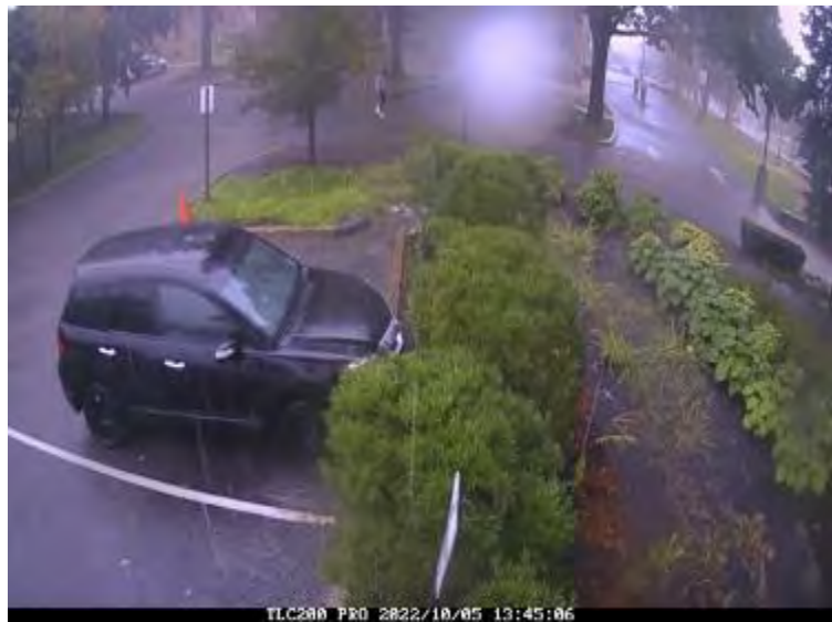
Infiltration basin treating runoff from parking lot at Providence College during heavy rain event. Inlet is working and berms are mostly containing flows. Overflow bypass appears to be functioning as intended. Photo: ASRI.
