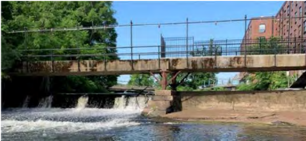
Downstream face of Pontiac Dam, Warwick, Rhode Island. Photo Credit: PRA.
