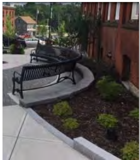
Flow Through Planter in Millbury, Massachusetts. Photo Credit: Town of Millbury .
