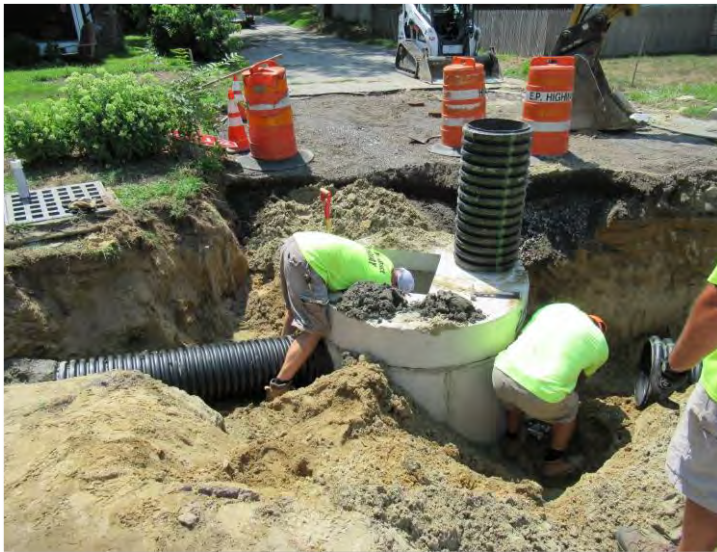
Retrofit installation on Willow Street in East Providence, Rhode Island. Photo Credit: East Providence, Rhode Island.
