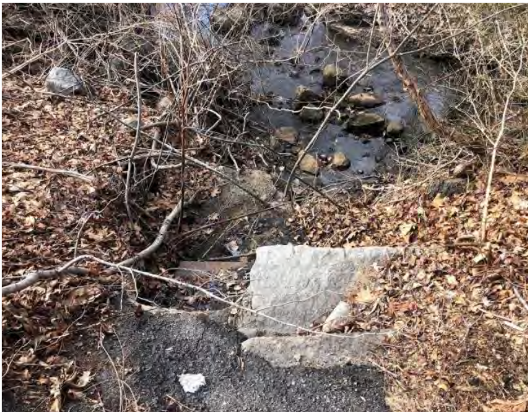
A paved swale directing untreated runoff to highly degraded section of the unnamed tributary to the Runnins River. Photo: East Providence, Rhode Island.
