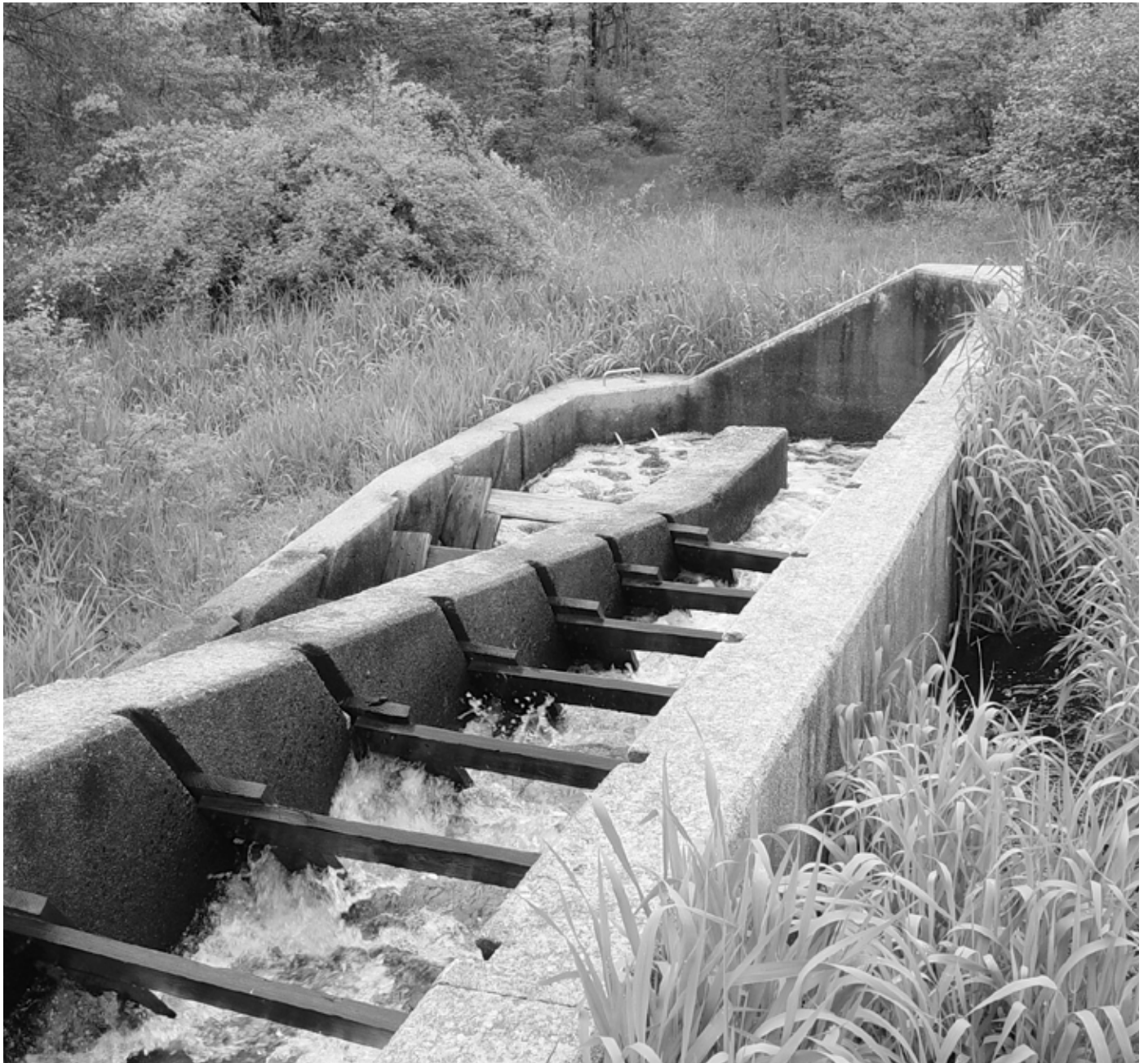
ABOVE Fish ladder at Bradford, R.I. provides access over a mill dam. BELOW Site of the Town Pond salt marsh restoration project in 1939, 1996, and 2008 – original pond, filled pond, and restored pond and marsh.
